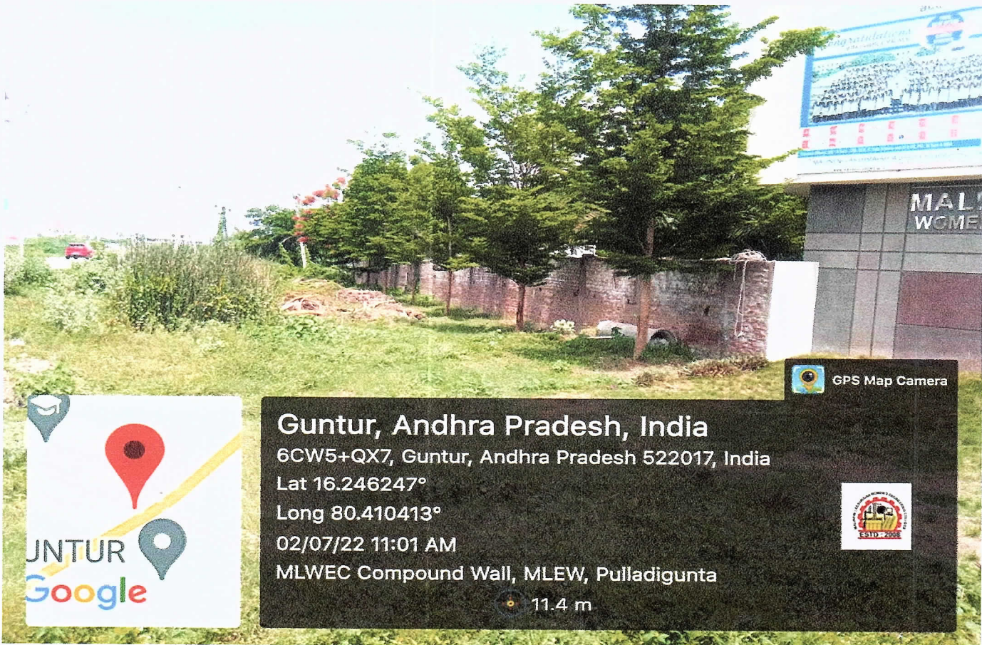
Compound Wall Of College
